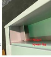
Wipe off any excess caulking. The top leg of the fascia is installed under the front lip of the gutter and then secured with a 3/4" tek screw and then the joint caulked to prevent leaking.
